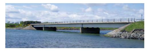
The current Waterside Bridge replaced a 7 span reinforced concrete bridge, built C1925, which was in an extremely poor condition by the mid 1980's due to the aggressive marine environment.
